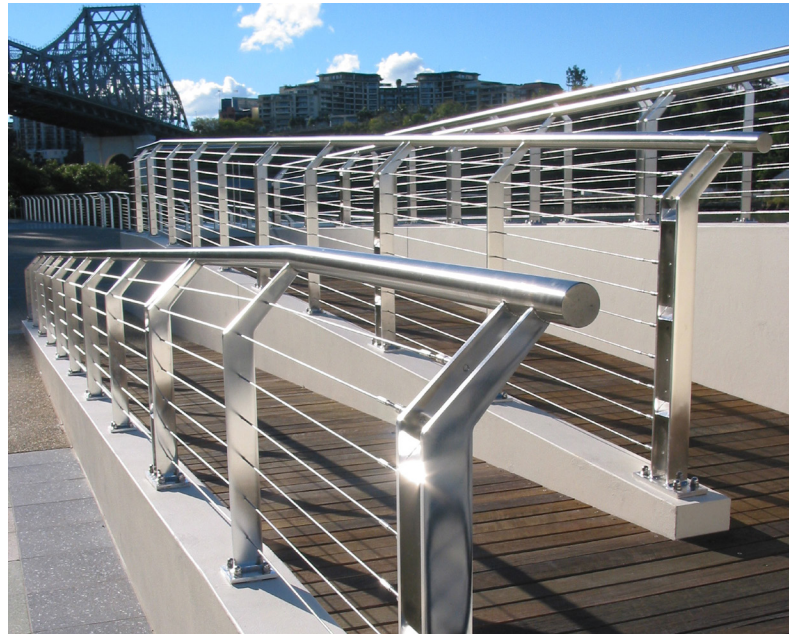
Holman Street, Brisbane: Example of successful use of stainless steel in a marine environment.
