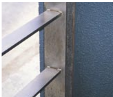
This photograph was taken a month after installation. Corrosion resulting from rough finishing technique is evident. Note also the crevices that are likely corrosion sites.
