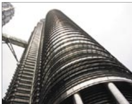
The Petronas Towers - a building with large side facets, clad with hyClad cambric patterned surfaces
