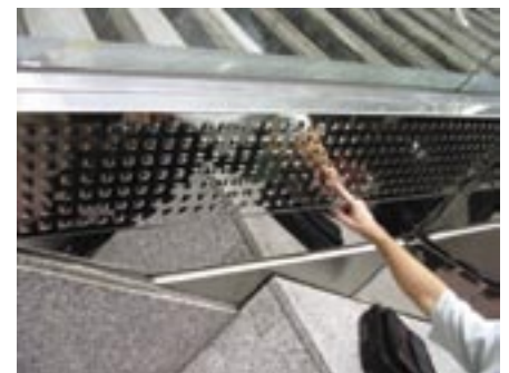
This decorative 2M finish was pressed into mirror polished sheet and while reflective, does not emphasise defects such as scratches, fingerprints and stains.
