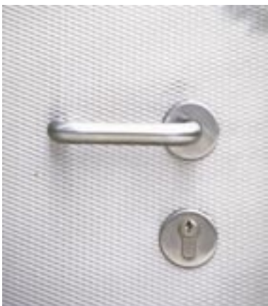
The door cladding provides strength as well as a bright appearance. Another example of strengthening is when a rigidised pattern is used for outdoor bench seating.
