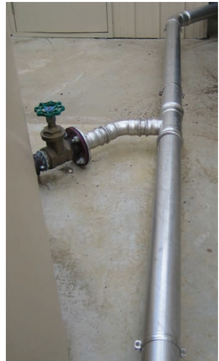
Casey Aged Care Facility, Heidelberg, Victoria
