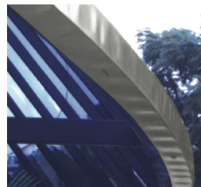
Ripples caused by welding practice.
